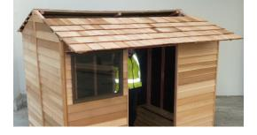
Step 14: Using 75mm tek screws, screw roof panels into end wall panels, (2 screws each end per panel), ensuring end of rafter lines up with centre of gable panel.
