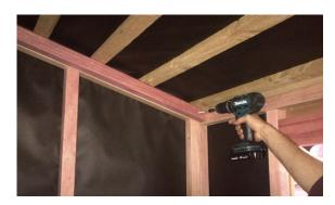
Step 15: Using 2 x 75mm framing nails, nail centre roof purlin to front and back top plate stiffeners. Predrill if necessary.
