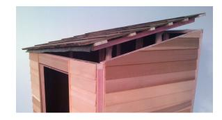
Step 14: Using 75mm tek screws, screw roof panel into end wall panels, (2 screws each end).
