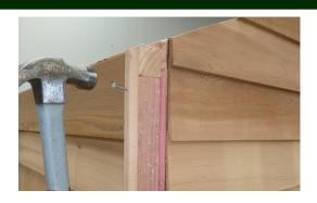
Step 12: Silicone and nail corner clashings on all corners as shown using 5 x bead nails per clashing.
