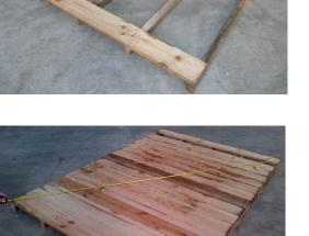
Step 2: Lay out remaining floor boards. Measure diagonals to ensure measurements are equal (i.e. floor is square). Rip down last floor board to suit gap, and nail off floor with 50mm flooring nails (10 nails per board).
