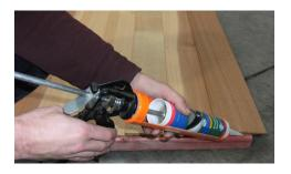
Step 7: Silicone and nail remaining beads on each panel. Screw panels together using 3 tek screws per join and 4 on the longer joins on gable end panels.
