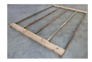
Step 2: Lay out remaining floor boards. Measure diagonals to ensure measurements are equal (I.e. floor is square). Rip down last floor board to suit gap, and nail off floor with 50mm flooring nails (10 nails per board).
