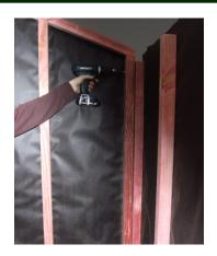
Step 6: Silicone edge of weatherboards on standing panel and nail on cedar beads with 5 x bead nails. (Refer to wall plan for correct beads).
