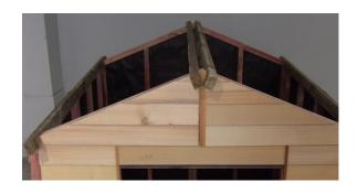
Step 14: Using a 75mm tek screw, screw bottom purlin to top plate centrally in shed.
