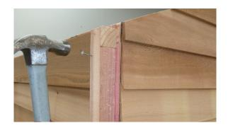
Step 12: Silicone and nail corner clashings on all corners as shown using 5 x bead nails per clashing.
