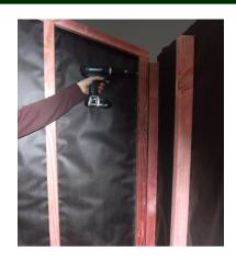
Step 6: Silicone edge of weatherboards on standing panel and nail on cedar beads with 5 x bead nails. (Refer to wall plan for correct beads). Make sure bead is properly sealed to avoid leaks. Note: On standard panels only, top of bead is bevelled to allow for slope of roof.
