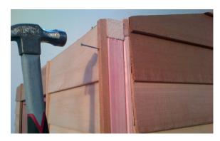
Step 12: Silicone and nail corner clashings on all corners as shown using 5 x bead nails per clashing. Note short clashings at the front, long clashings at the rear.
