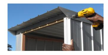
Step 3: Line up ribs on the roof with ribs on the walls. While someone holds the Front Plate straight, predrill using a 3.5mm drill bit and screw the roof to Top Plate using one 55mm Roofing Screw on each rib. (Outside ribs do not need to be fastened). Repeat at the back. Note: a string line can be used to make this easier.
