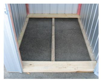
Step 3: Lay out remaining Floor Boards. You may need to cut the last Board to correct width using Skill saw. Nail in each Floor Board, two 50mm nails each end and two into Floor Joist.
