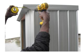
**Step 3:** Line up ribs on the roof with ribs on the walls. While someone holds the Front Plate straight, predrill using a 3.5mm drill bit and screw the roof to Top Plate using one 50mm Roofing Screw on each rib. (Outside ribs do not need to be fastened).
