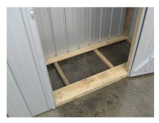
Step 3: Lay out remaining Floor Boards. You may need to cut the last Board to correct width using Skill saw. Nail in each Floor Board, two 50mm nails each end and two into each Floor Joist.
