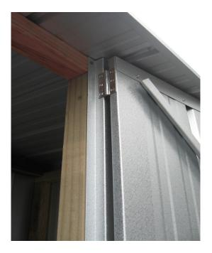
**Step 3:** Close door and check it fits correctly. If not, drill out rivets and make necessary adjustments. Fit remaining rivets to all three hinges.
